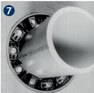
**7** Repeat tightening after approx. 2 hours. Especially for LINK-SEAL® Type LS 500 up to LS 700 it might be necessary (depending on the installation conditions such as annular space, temperature, etc.) to tighten again for several times.
