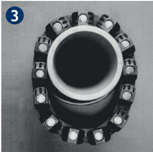
**3** Check to be sure bolt heads are facing the installer. Extra slack or sag is normal. Do not remove links if extra slack exists. Note: On smaller diameter pipes, links may need to be stretched.
