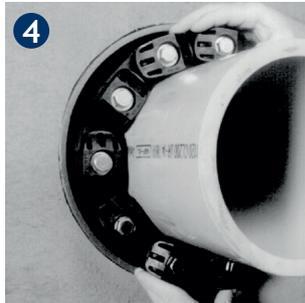
**4** Slide belt assembly into annular space. For larger size belts, start inserting LINK-SEAL® modular seal assembly at the 6 o'clock position and work both sides up toward the 12 o'clock position in the annular space.
